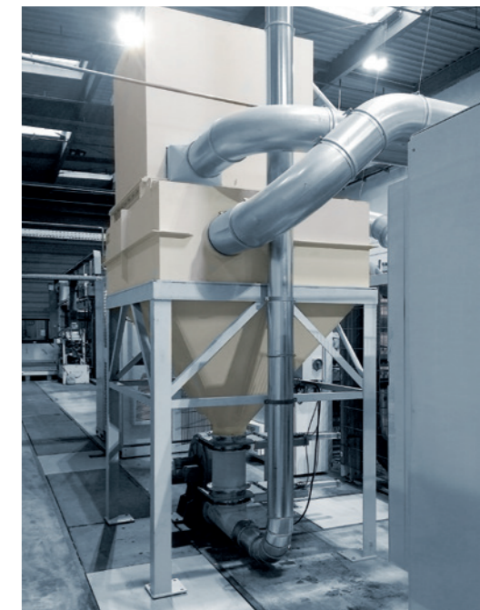
KELVA filter/fan unit AFF-I42 with waste handling connected to a central system
